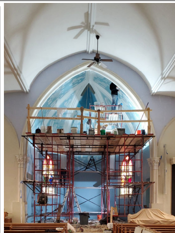
Status of Sanctuary Renovation as of Wed, Apr 17.
